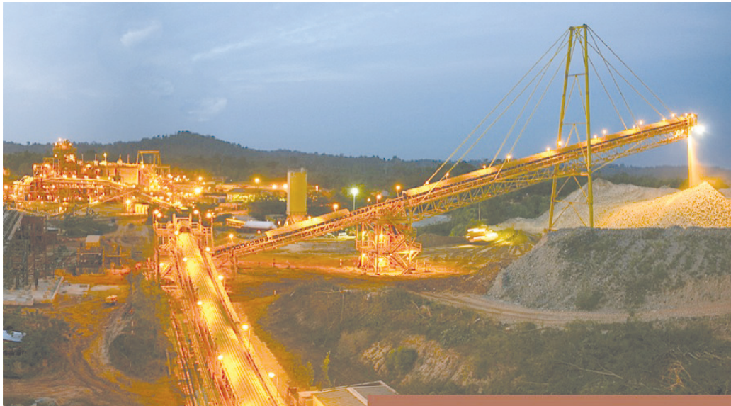
Crushed ore stock pile at Damang Gold mine in Ghana. (Image courtesy of Gold Fields)
